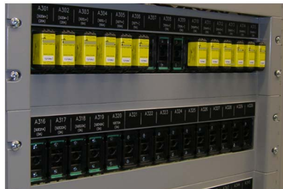
Figure 8 Dead-front fuse assemblies mounted on a rack for easy access to the fuses.
