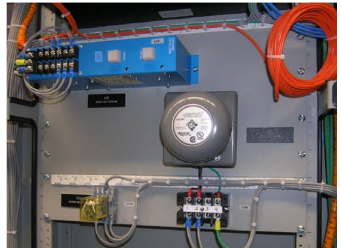
Figure 11 Equipment mounted on a blank panel attached to the rear of a rack.
