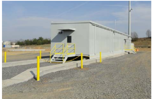
Figure 25 Medium sized control building at a 500kV substation consisting of Command Module #1, one Telecom Module #1, one P&C Module #1, and an End Cap Module.
