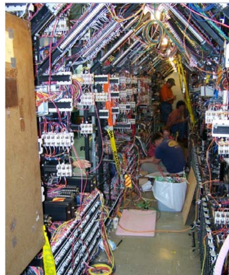
Figure 2 Electricians in close proximity to live terminals at an older station.
