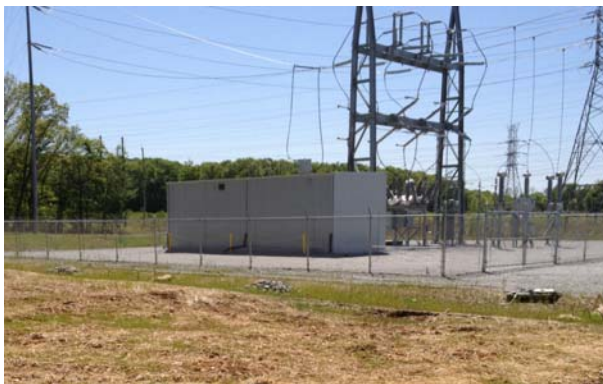
Figure 24 Small control building at a substation consisting of a Command Module #2, a Combined P&C and Telecom Module, and an End Cap Module.
