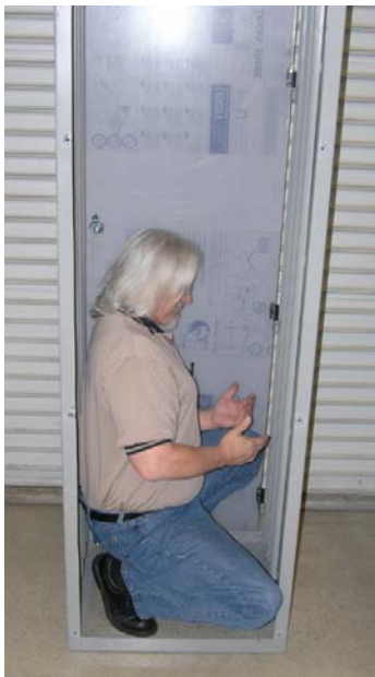
Figure 3 Shows two views of an employee simulating work in a 24" cabinet. Note: If equipment was installed in this cabinet, then working spaces would be further reduced. Also note cabinet threshold by employee's shoe.
