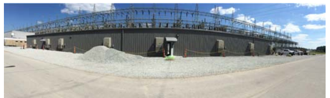
Figure 26 Large control building at a 161kV generating site consisting of Command Module #1, two Telecom Modules #1, four P&C Modules #1, and an End Cap Module.
