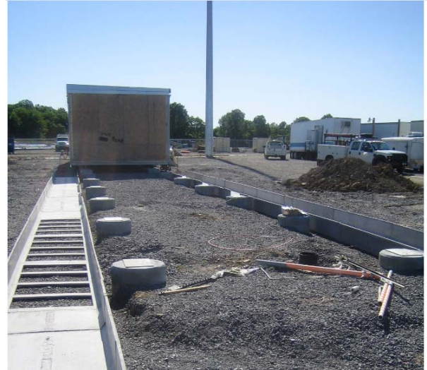
Figure 27 Control building during assembly showing foundations and cable trenches along the sides of the building. The Command Module with its temporary plywood wall is shown in the distance resting on its foundation.
