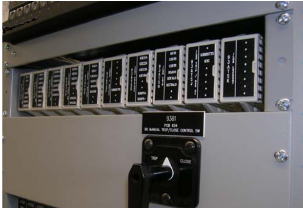
Figure 9 Test switch assembly containing ten test switch modules giving a total of 80 test points in a 2RU frame mounted below a relay. Note: TVA nameplates are affixed to test switch doors for identification of test switches.
