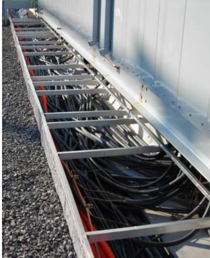
Figure 28 Cable trench showing removable metal frame to support covers. Note: Gutter downspouts will be provided with an extension over the cable trench when construction is complete.
