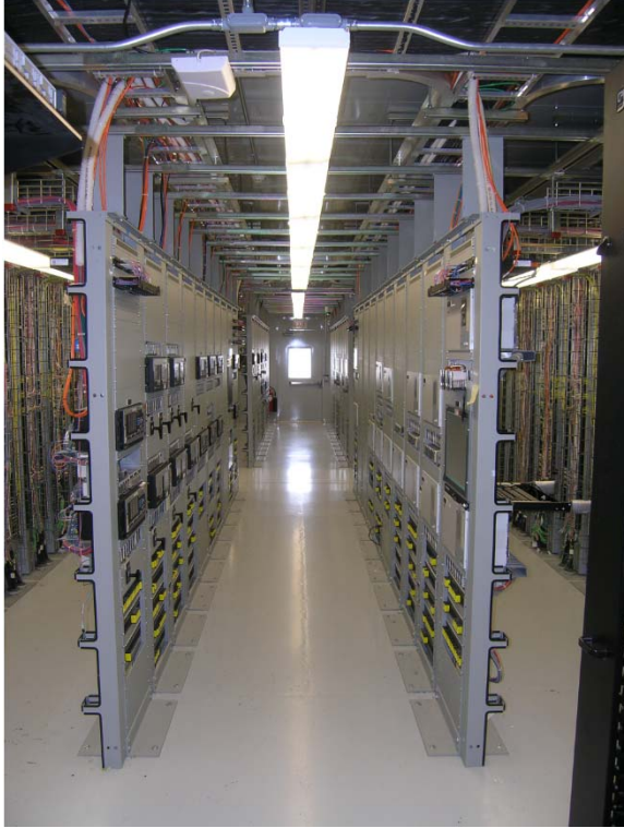
Figure 15 Photograph through the control building showing the live front and dead front hallways in two consecutive P&C modules. Note: The photo also shows the cross streets between the modules.
