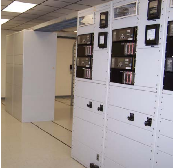
Figure 1 1990s vintage relay cabinets at TVA.
