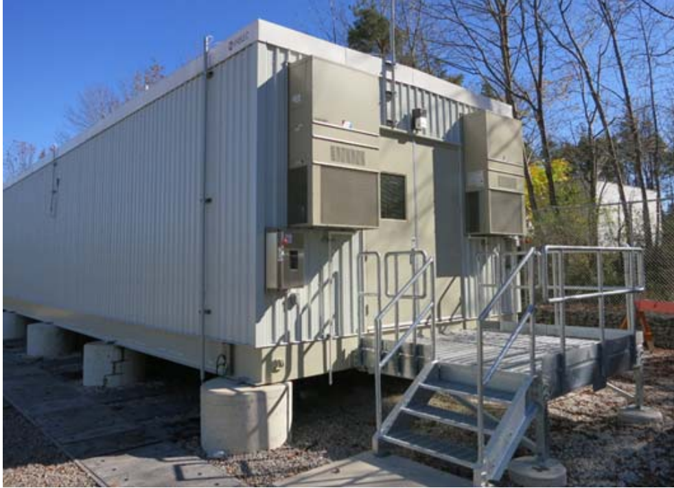
Figure 1 - Drop-In Relay/Control Room
